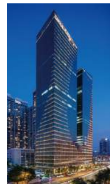
Example of managed property (Capital Place)
