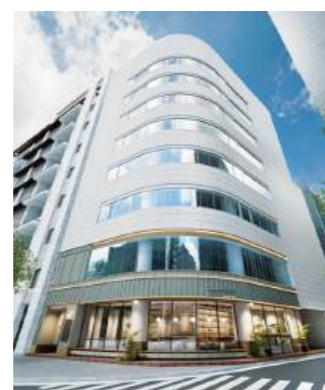
Yotsuya-sakamachi renovation project
